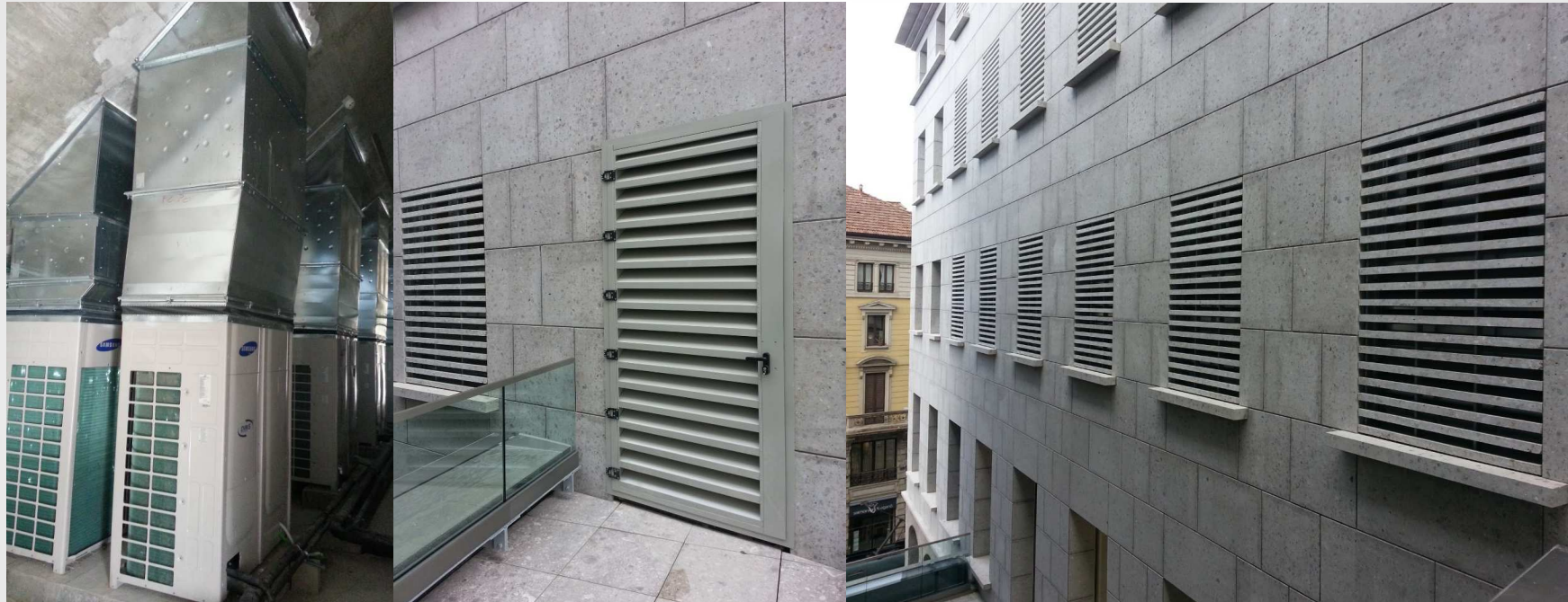
Shopping Center Via Torino – Milan Sound attenuators, Acoustic Grilles
